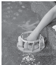
Turn filter cartridge counterclockwise to unscrew.
